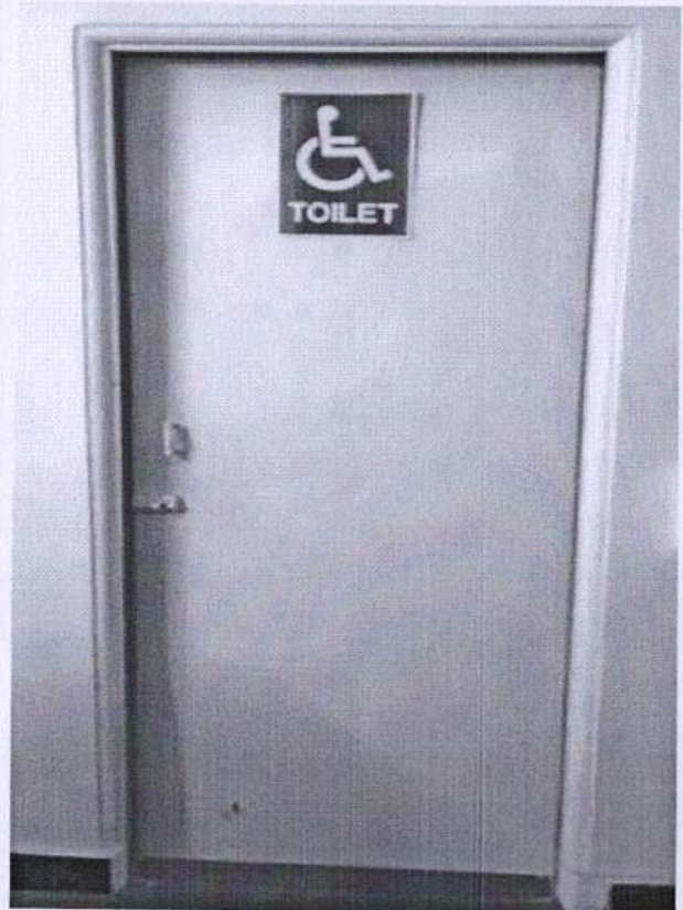
REST ROOM FOR PHYSICALLY CHALLENGED
